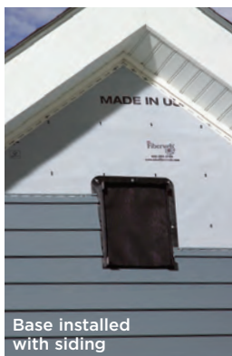
Vent Cap installed after siding is finished
